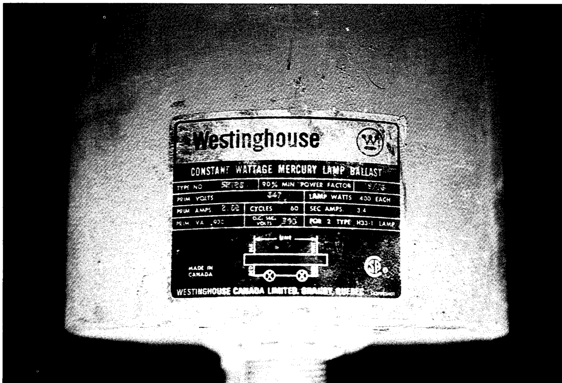
8d. Close-up of Photo 8c. The date code, G/73 (located below the word "BALLAST"), indicates that the ballast was made in July 1973, and contains PCB-filled capacitors.
