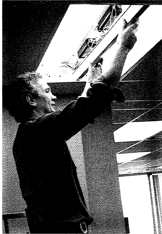
1b. The heat shield is removed, exposing the lamp ballasts.
